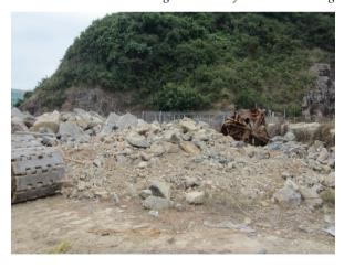
**Photo 4** -Tarpaulin sheets to cover open stockpiles to prevent dust generation were absent from the construction site.
